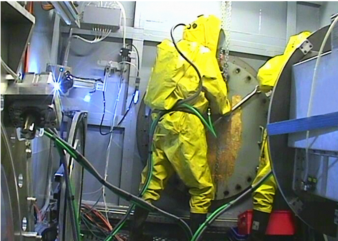
Mounting of Inspection System in habitat
