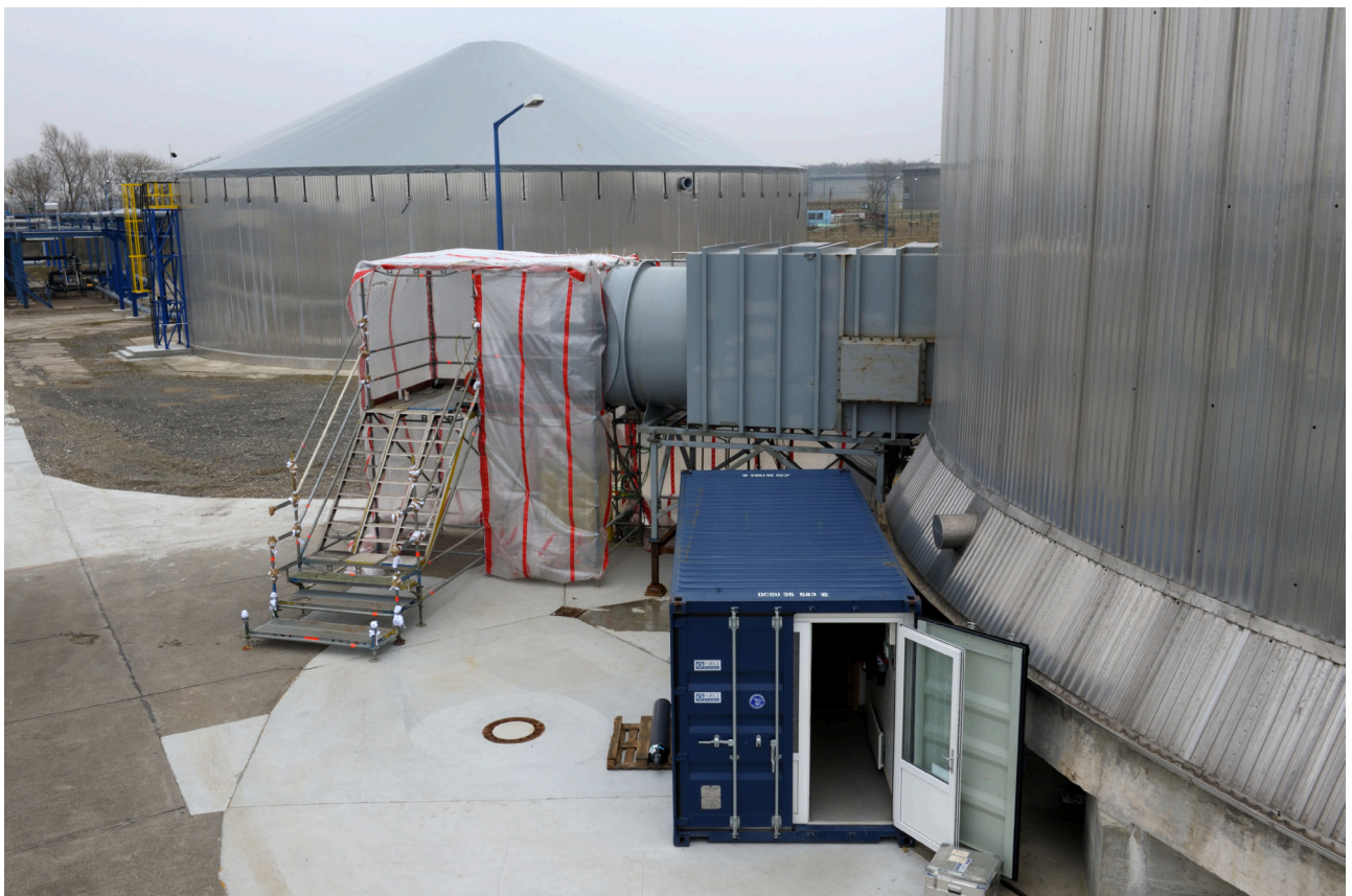
Control room and shop in front of habitat
