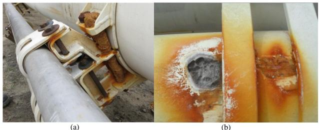
(a) (b) Figure 7: (a) Large variation in condition of bolts for clamps. (b) Excessive corrosion at
