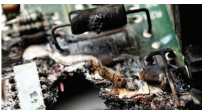
ELECTRICAL SAFETY TEST
