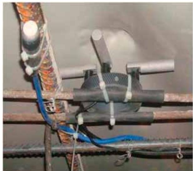
CorroWatch and ERE 20 fixed to reinforcement in tunnel
