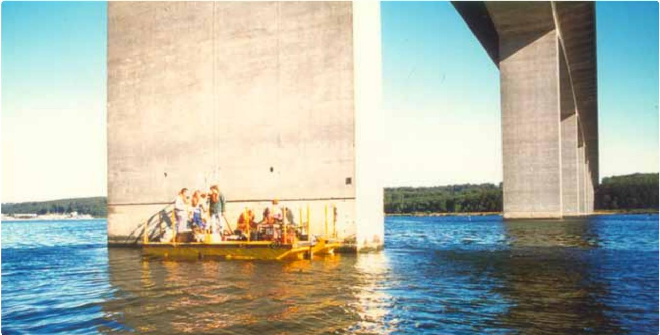
*Installation of corrosion sensors in concrete pillar of marine bridge*
