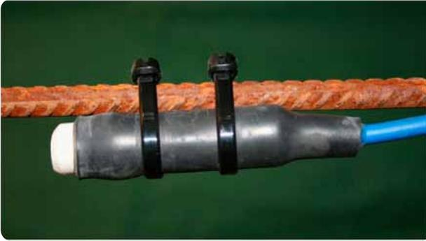
ERE 20 fixed to reinforcement before pouring of concrete
