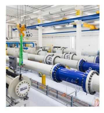
All closed loops are connected to a transmission pipeline, allowing a fast supply of gaseous flows like air, natural gas, biogas and mixtures with hydrogen within an hour.
