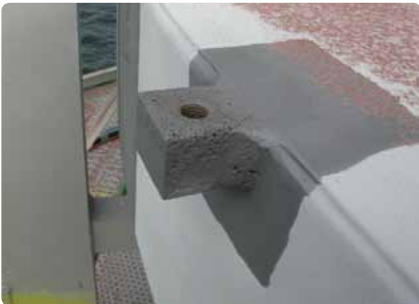
Painting inspection - Offshore windturbines
