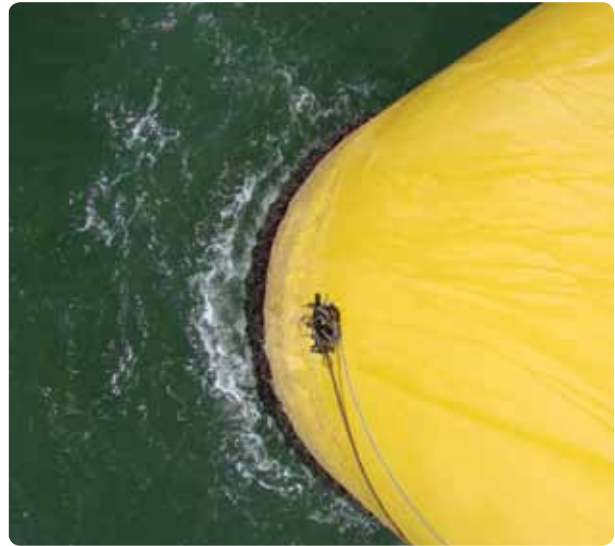
Ultrasonic inspection of transition piece from the outside
