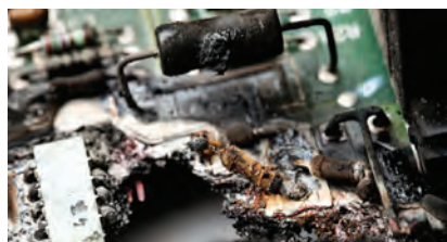
ELECTRICAL SAFETY TEST
