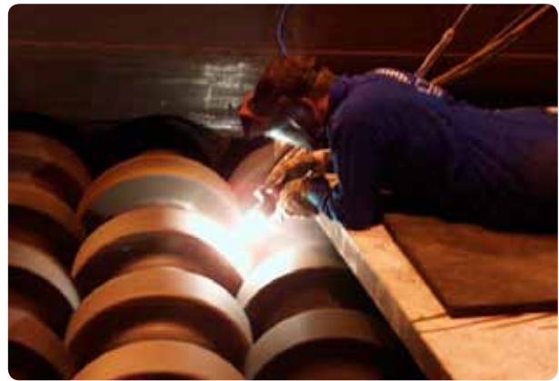
Repair by thermal spraying of large and costly application on-site
