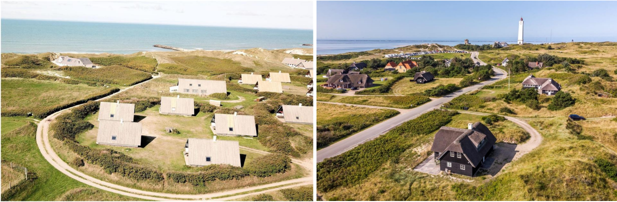
Figure 1 Examples of Danish summer houses / cottages behind and in the sand dunes at ‘Vesterhavet’ (The North Sea). Pictures from [8-9].
