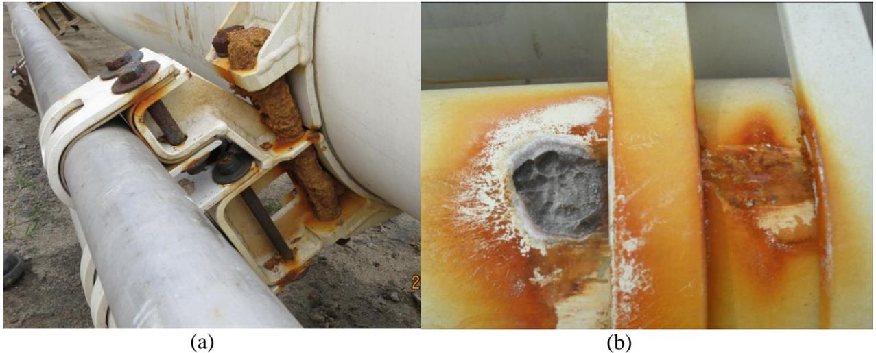
Figure 7: (a) Large variation in condition of bolts for clamps. (b) Excessive corrosion at clamp.
