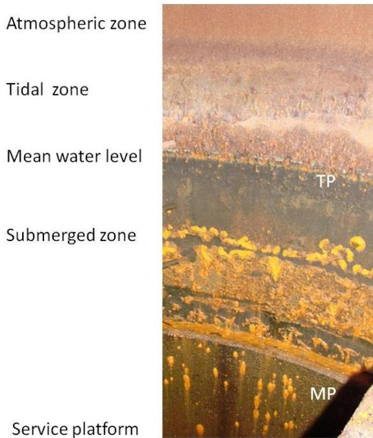
**FIGURE 5:** Appearance of corroded surface inside a monopile.
