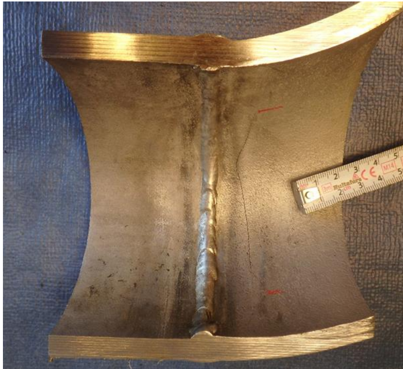
Crack length ~85 mm, up to 0.2 mm wide.
