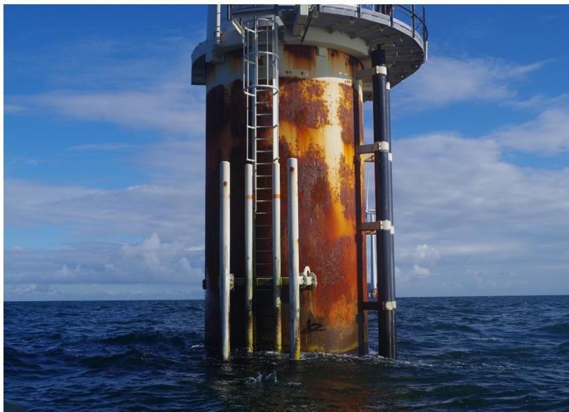
**Figure 4: The thin 350  $\mu\text{m}$  coating system after 14 years of service (2016). Extensive corrosion and almost complete loss of coating is observed.**
