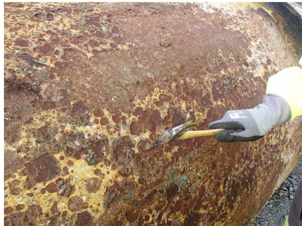
**Figure 9. Corrosion on jacket leg in an area that originally had been shielded. The corrosion depth is 2-3 mm.**
