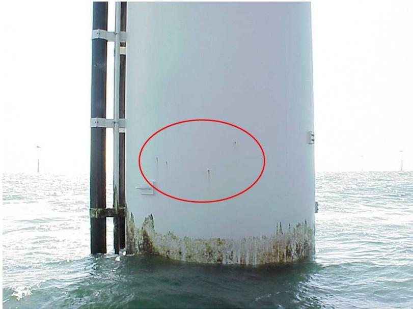
**Figure 2: The thin 350 µm coating system after 2 years of service (2004). Pinpoint rusting (Rust Grade 9-P, SSPC-VIS 2) has started.**
