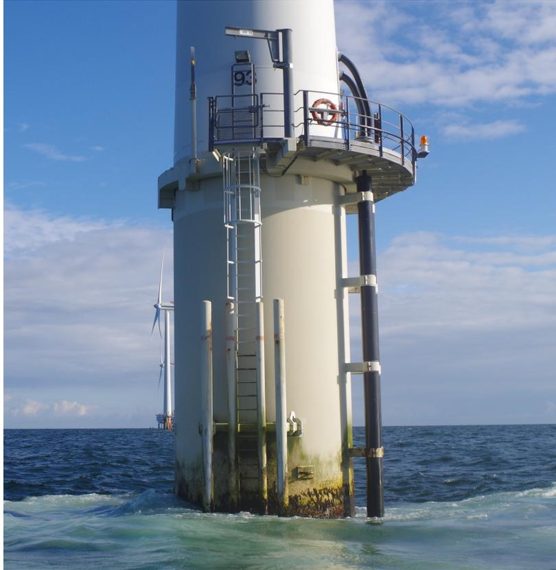
**Figure 5: The 1000  $\mu\text{m}$ , 2-coat solvent free epoxy coating system after 14 years of service (2016). Completely intact coating system and no visible corrosion is observed on the TP.**
