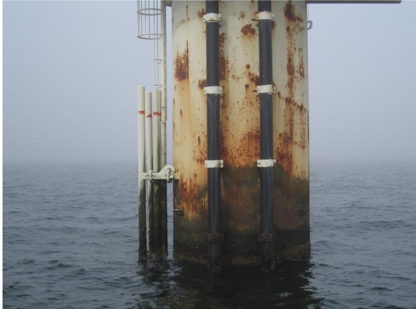
**Figure 3: The thin 350  $\mu\text{m}$  coating system after 12 years of service (2014). Extensive corrosion and coating breakdown is observed.**
