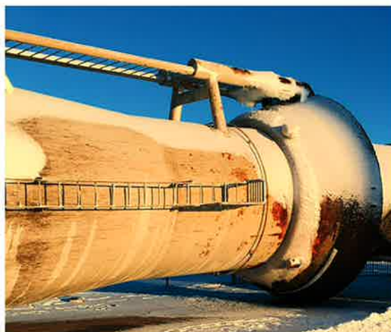
Fig. 4: This image shows a decommissioned TP from Yttre Stengrund Wind Farm, Baltic Sea, Sweden, after more than 15 years of service. The splash zone area has been attacked by ice, other impacts and general wear. The area above the splash zone is in fairly good condition. The brackish, low-saline water and the cold climate of the Baltic Sea may have contributed to the lesser corrosion.
