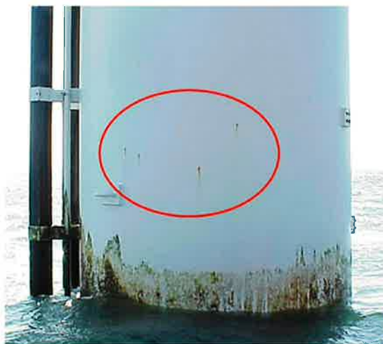
Fig. 2: At the Horns Rev 1 (HR1) facility, pinpoint corrosion is noted on TPs painted with the lean two-coat epoxy system, Photos, Figures 2-4, courtesy of FORCE Technology
