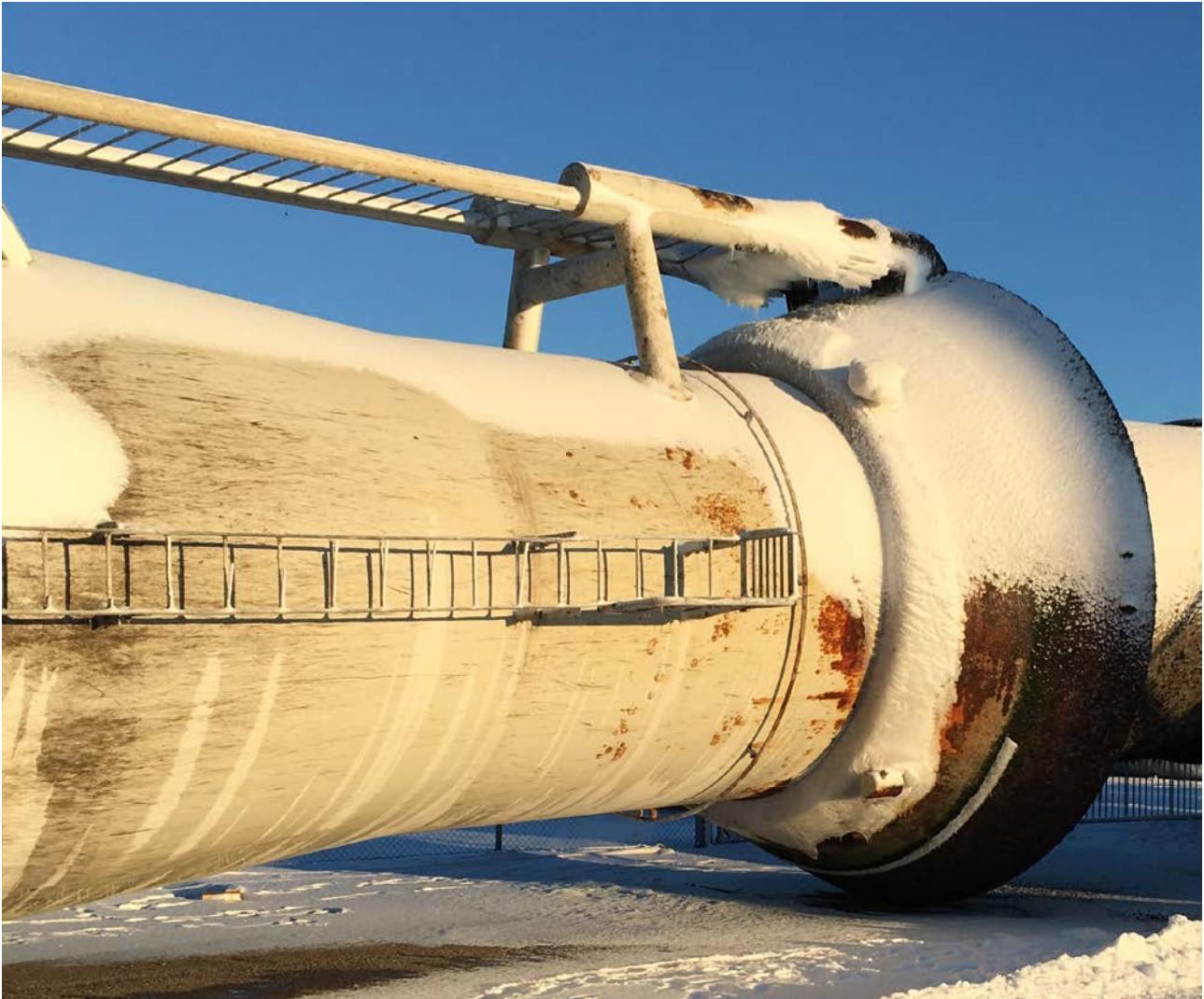
Figure 4. Decommissioned TP from Yttre Stengrund Windfarm, Baltic Sea, Sweden, after more than 15 years of service. The splash-zone area is attacked from ice and other impacts and general wear. The area above the splash-zone is in fairly good condition. The brackish, low saline water and the cold climate of the Baltic Sea may have contributed to the lesser corrosion.
