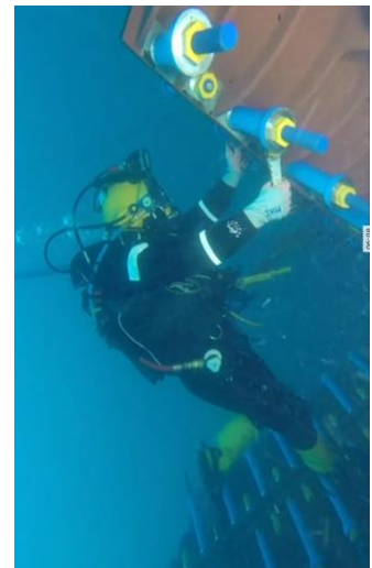
Clamp installation on oil rig. Source: ing.dk
