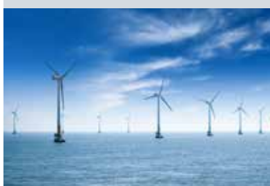
Fast Track 11: Optimizing surface protection system of wind turbine towers
