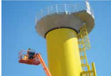
Fast Track 2: Corrosion protection of monopiles
