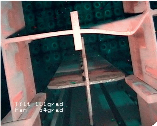
Visual inspection of a core grid in a reactor vessel
