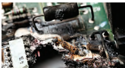
ELECTRICAL SAFETY TEST
