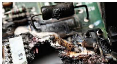
ELECTRICAL SAFETY TEST
