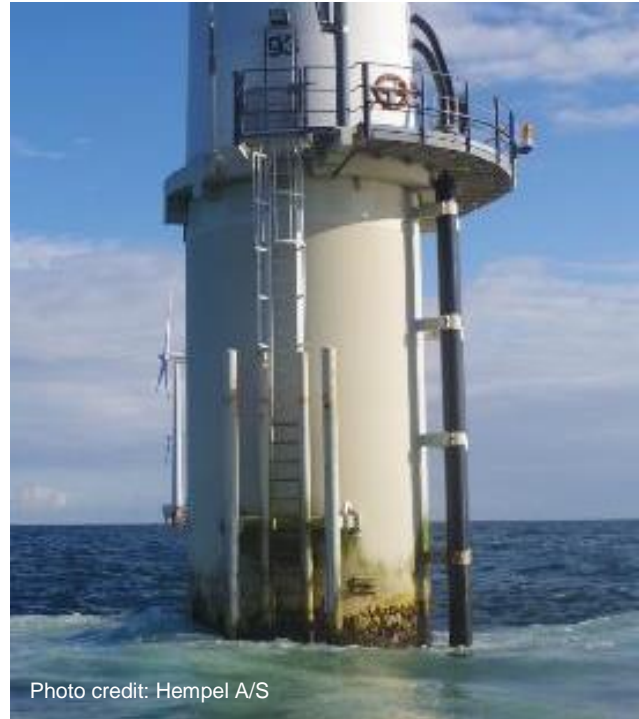
Figure 2: Two-coat epoxy system in 1000 µm (DFT) – no NORSOK approval.
