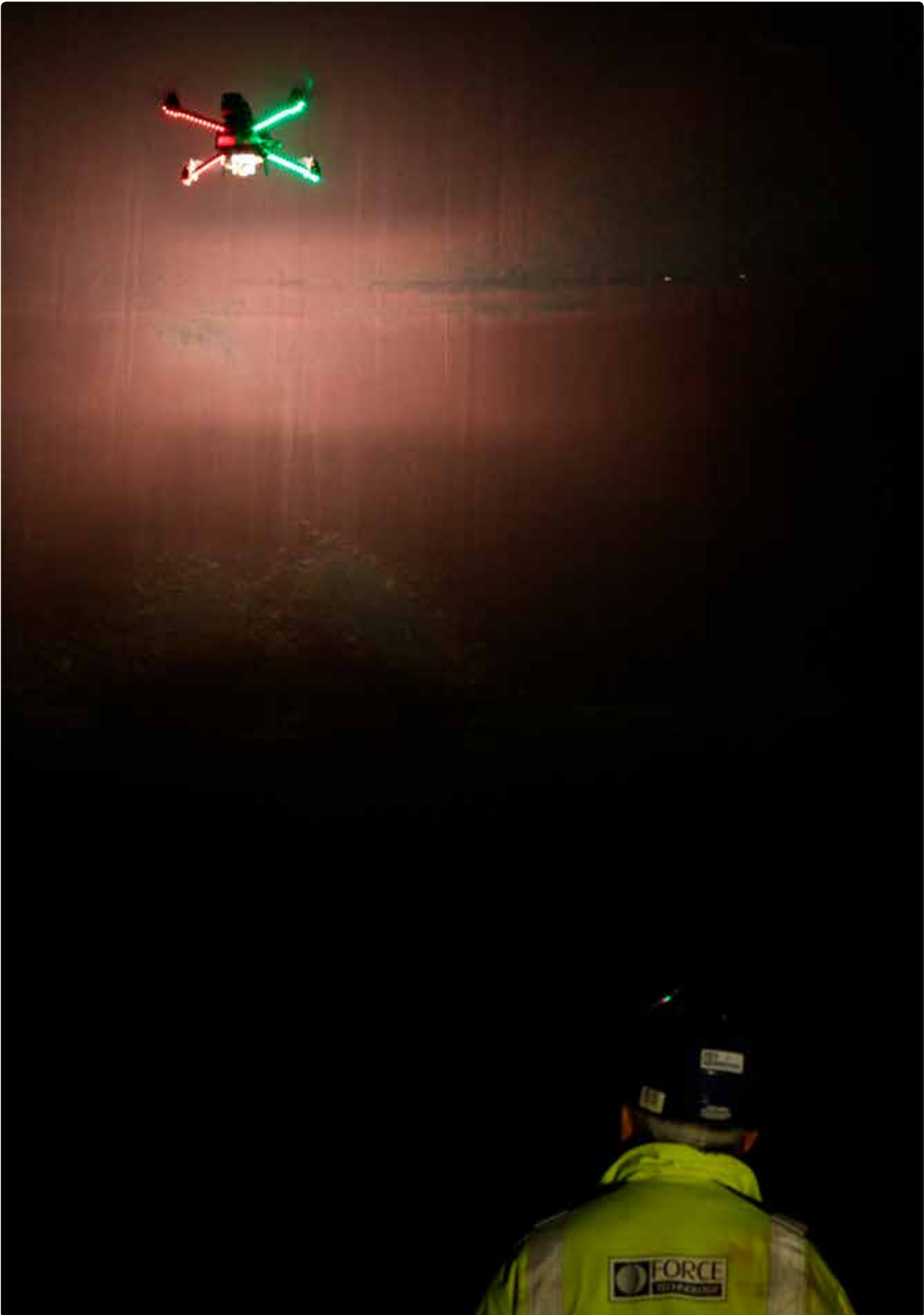
Drone inspection of an underground storage tank.
