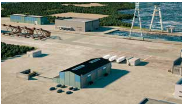
The infrastructure is ideal in relation to shipping and handling large structures.
